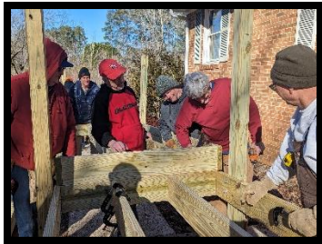
January "Ramp It Up" Build
